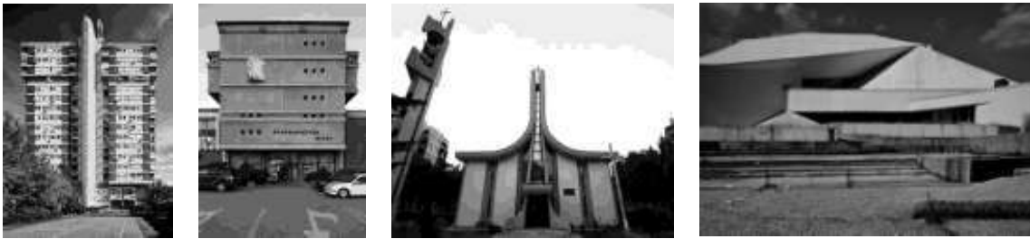
Figure 5: S. Gjurikj, B. Micevski's Catholic Cathedral , D. Dimitrov's Residential Tower , T. Dimitrov's Museum of natural history and Biro71's Macedonian Opera and Ballet House . Source: www.marh.mk/betonsko-skopje/ .
