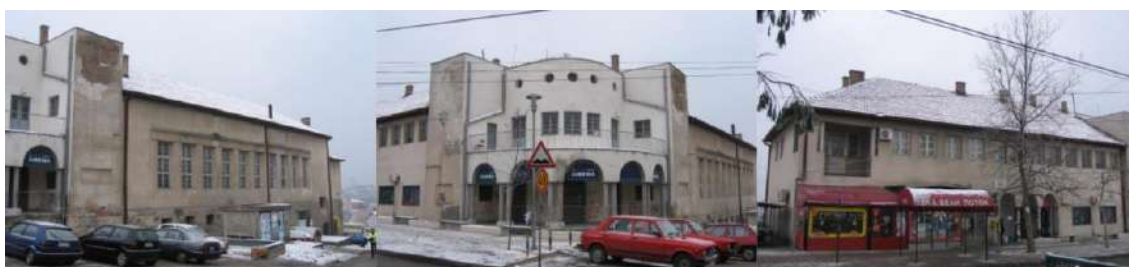
Figure 4: In the middle: The part of the Cooperative Home in Beli Potok / Belgrade that has been renovated. Left and right: Side wings with great conversion and reactivation capabilities. (Source: from the author's archive)
