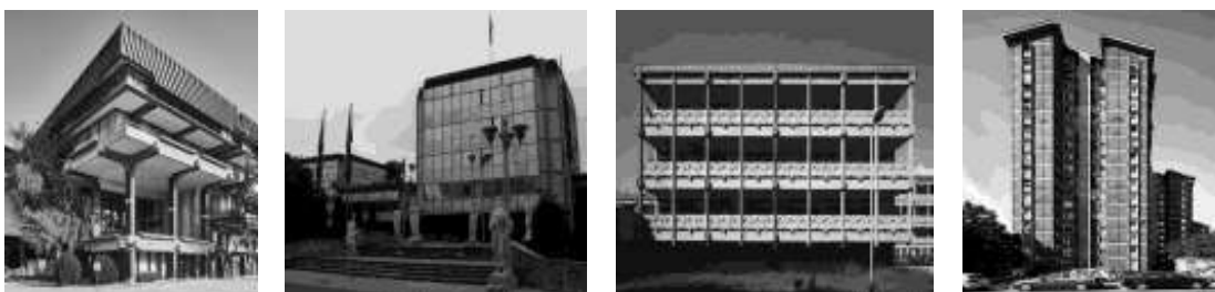
Figure 7: B. Čipan, MANU, P. Mulićkoski’s National and University Library, Central Committee of the League of Communists and B. Micevski Kapištec Tower. Source: www.marh.mk/betonsko-skopje/ .
