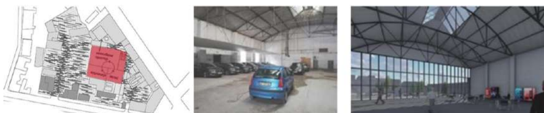
Figure 6: Proposal of the revitalization of a former warehouse – intervention position within the complex (left), current state (middle), a proposal of revitalization (right)
