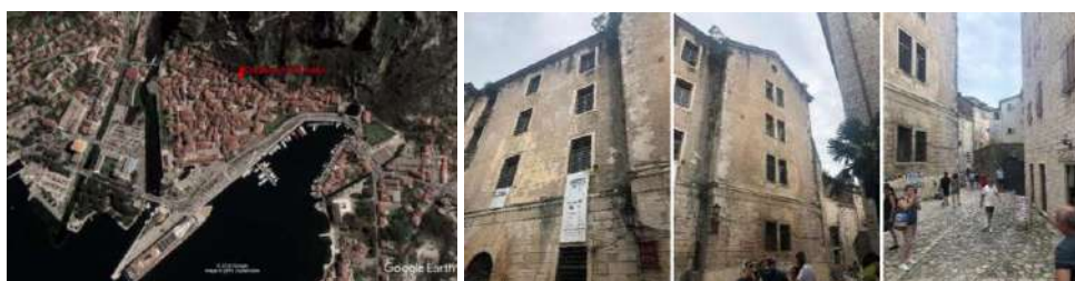
Figure 3: Urban heritage of the Old Town Kotor – Ministry of Culture of Montenegro (2018). “Feasibility study for the valorisation of the location of the Prison building in the Old Town of Kotor”.
