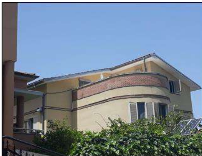
Figure 2. Exterior view of the masonry building
