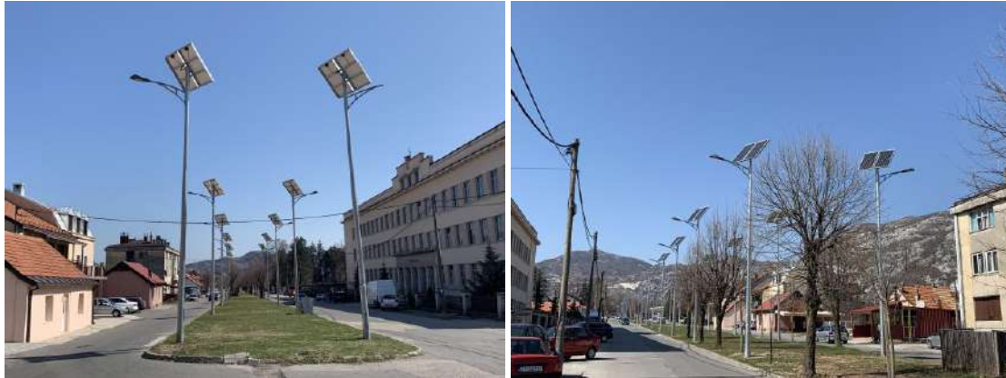
Figure 3 Solar street-lighting in the Boulevard of Montenegro Heroes, Cetinje, Montenegro (photo G. Radović)
