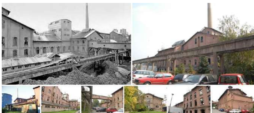
Figure 1: The mashine room in time of the full production (upper left) and current state of the Sugar factory
