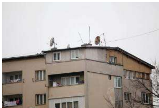
Source: Gazeta Zeri –Illegal construction loft roof your land”
