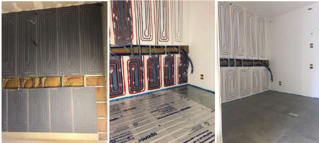
Figure 3: Construction sequence of radiant floor and walls.
