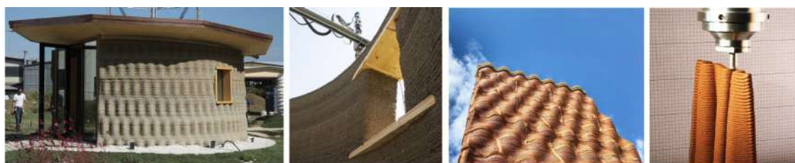
Figura 3: Stampa 3D per l'involucro - Gaia (© WASP), Sistema costruttivo a blocchi IAAC (©G.Paparella, ©Pylos, a project of IAAC, developed within the OTF program, by Sofoklis Giannakopoulos)
